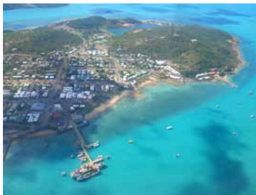
Horn Island jetty
