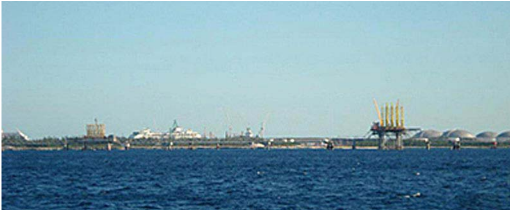
Freeport—Borco Oil Terminal
