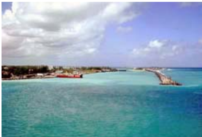
Arawak Cay—West Breakwater
