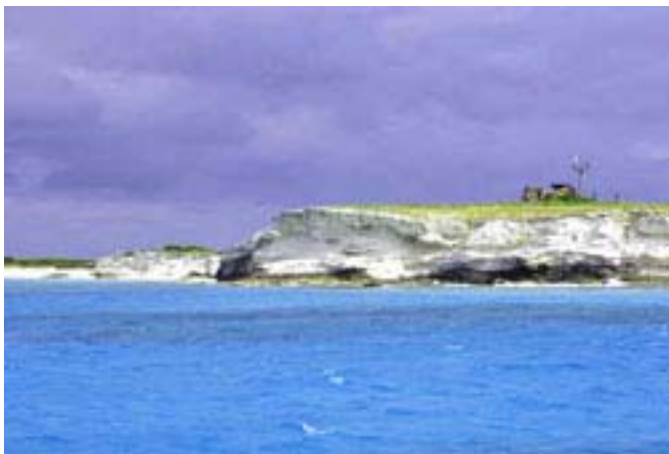
Big Sand Cay Light (right side next to old fallen light)
