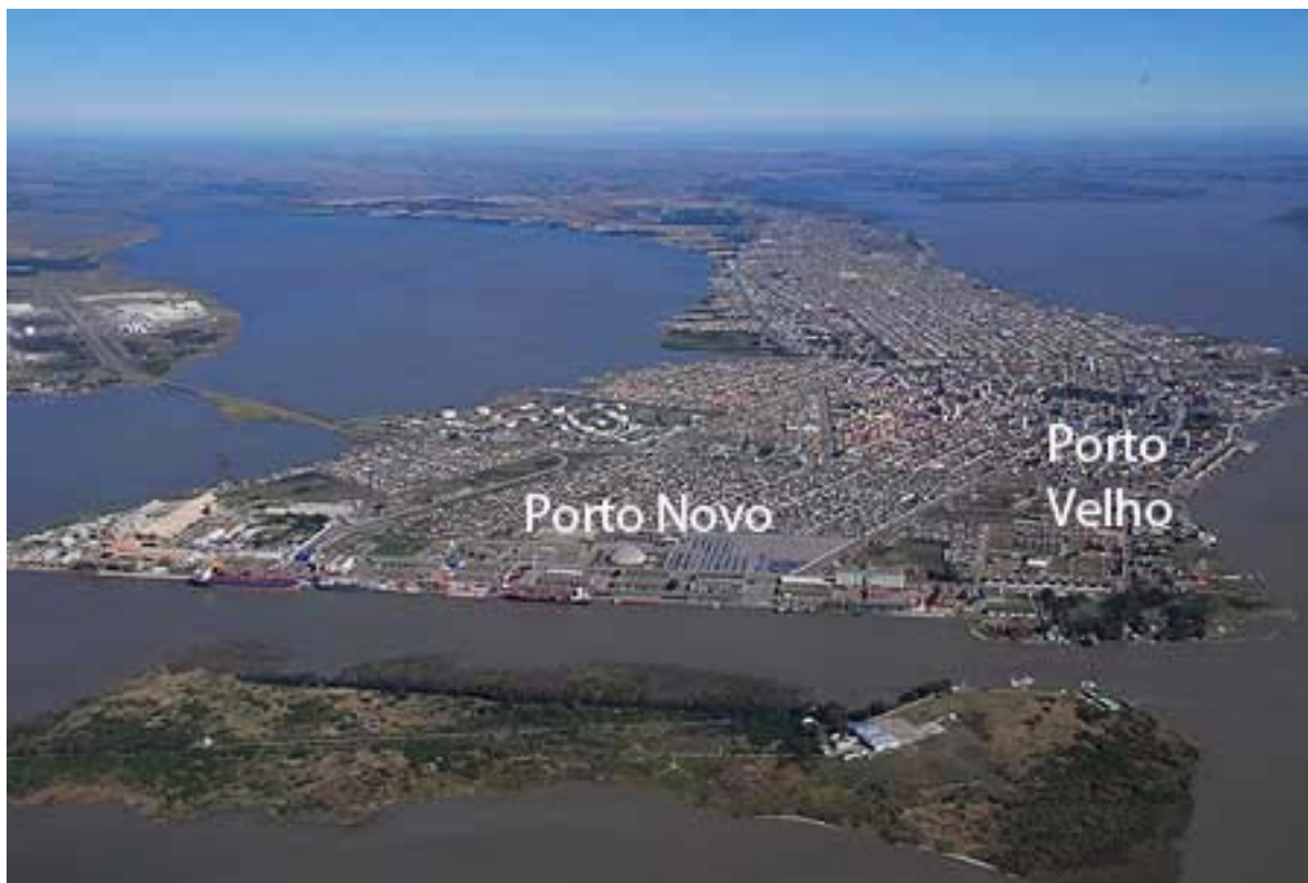
Aerial view of Rio Grande
