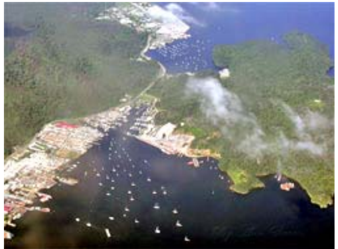
Chaguaramas Terminal Wharf (center)
