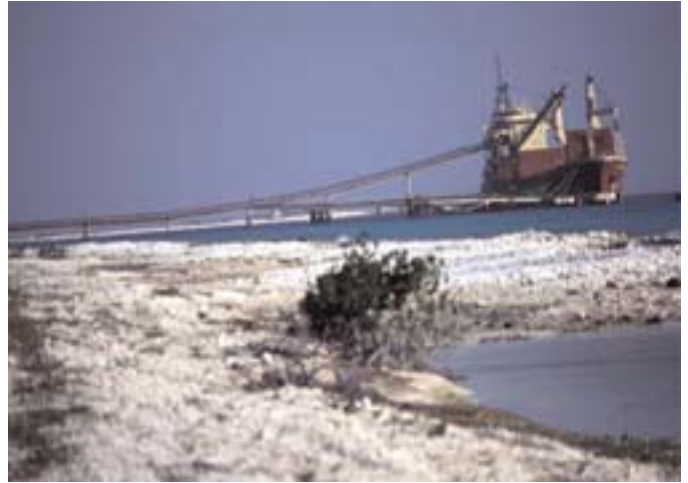
Zoutsteiger Pier (for bulk salt)
