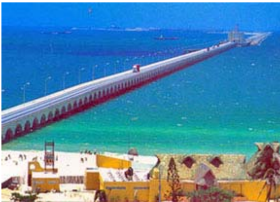
Progresso—Terminal Remota Pier
