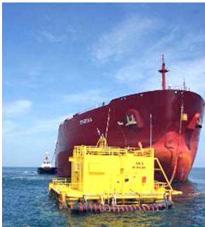
Covenas Tanker Loading Unit (TLU-2)
