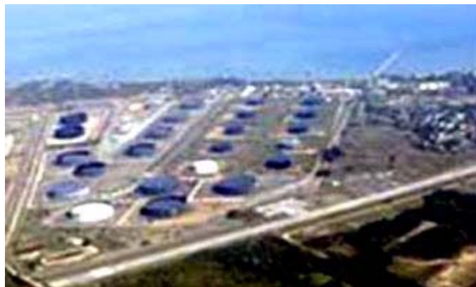
Covenas Tank Farm
