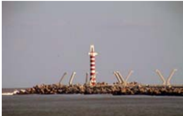
Coatzacoalcos Entrance Light on the breakwater
