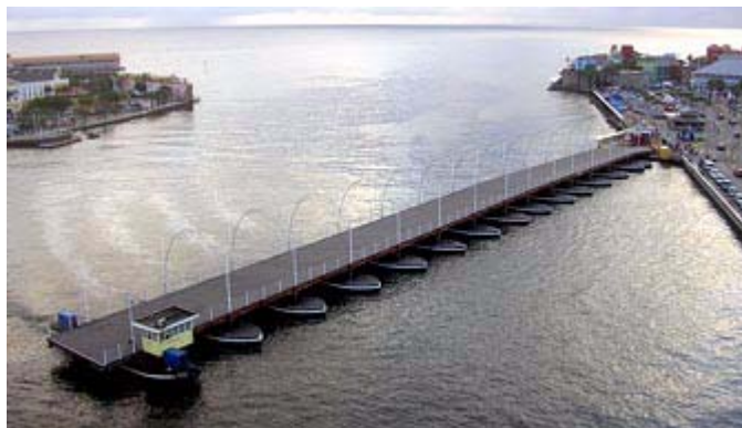
Queen Emma pontoon bridge
