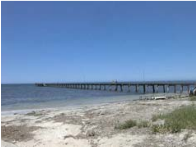
Marion Bay Jetty
