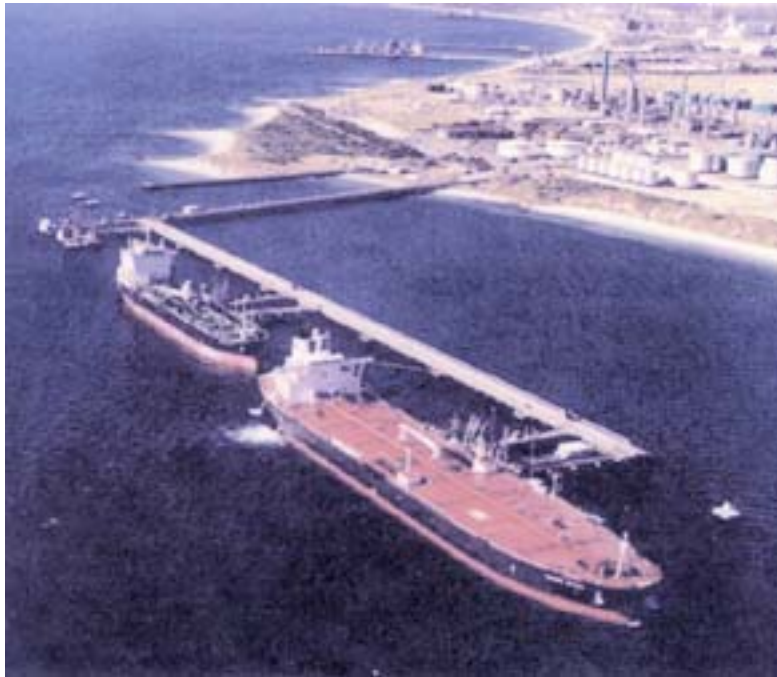
Courtesy of Fremantle Port Authority Fremantle—Outer Harbor—Kwinana Oil Refinery Jetty
