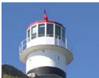
Cape Point Disused Light Structure
