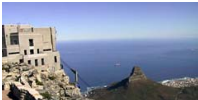
Upper Cable Station (Table Mountain)
