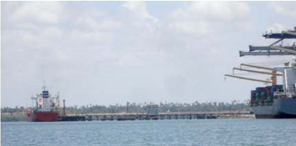
Dar es Salaam Harbor—Kurasini Oil Jetty
