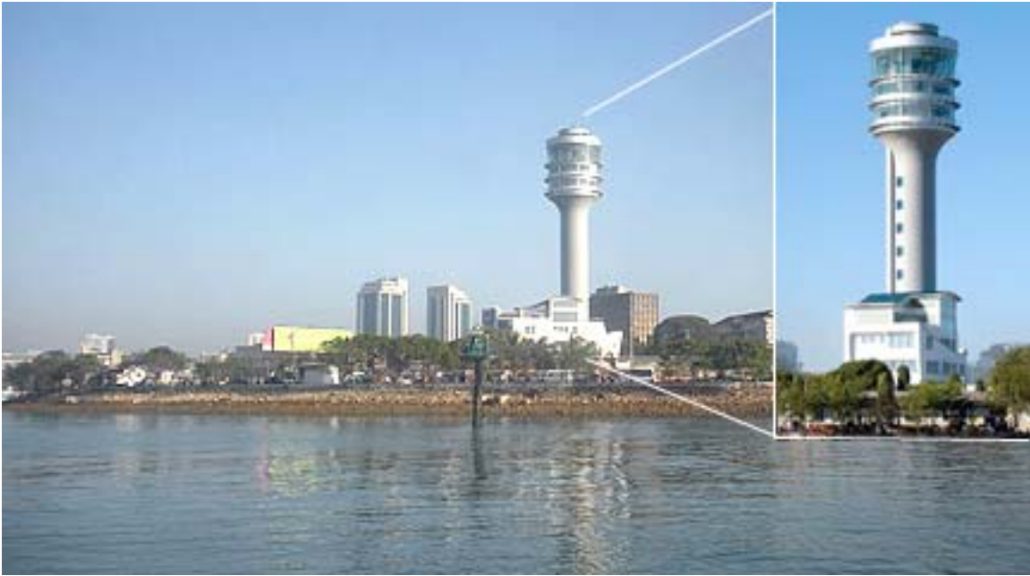
Dar es Salaam—Harbor Approach with Vessel Traffic Control Tower
