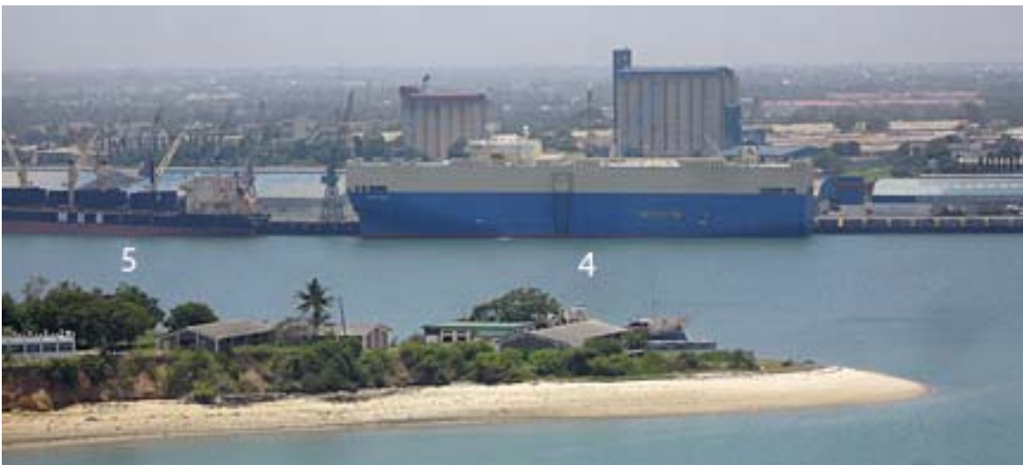
Dar es Salaam—Berths 4 and 5
