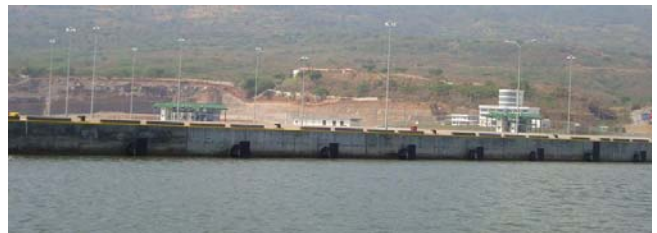
Puerto La Union Wharf from SE
