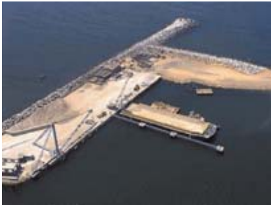
Ensenada Petroleum Terminal
