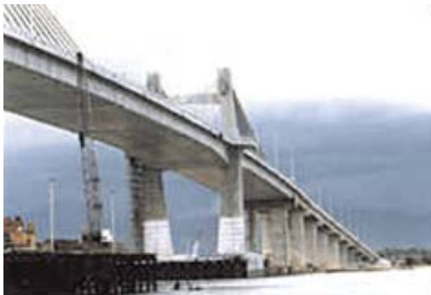
The Mandaue-Opon Bridge (Mactan Bridge)
