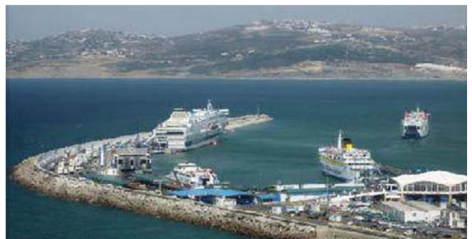
Port of Tanger Breakwater from W
