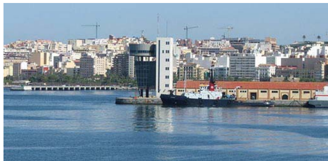
Ceuta Harbor Control Tower
