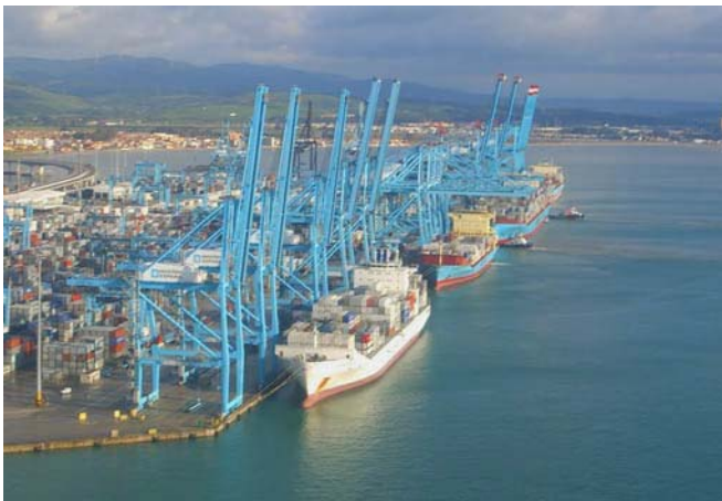
Maersk Container Terminal
