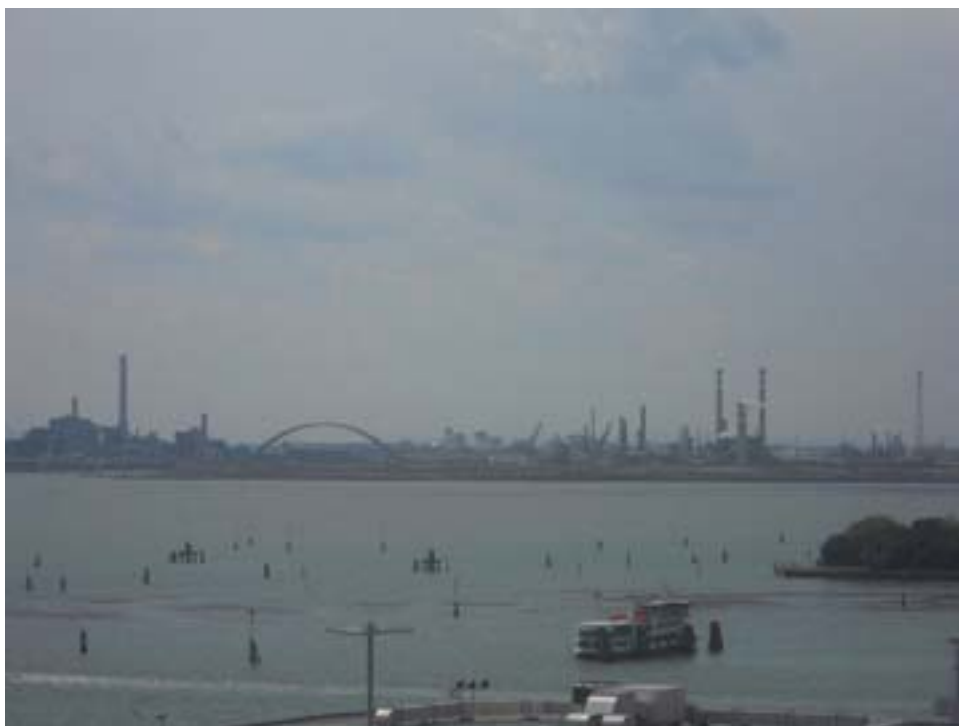
Overhead pipeline at entrance to Canale Industriale Sud from E
