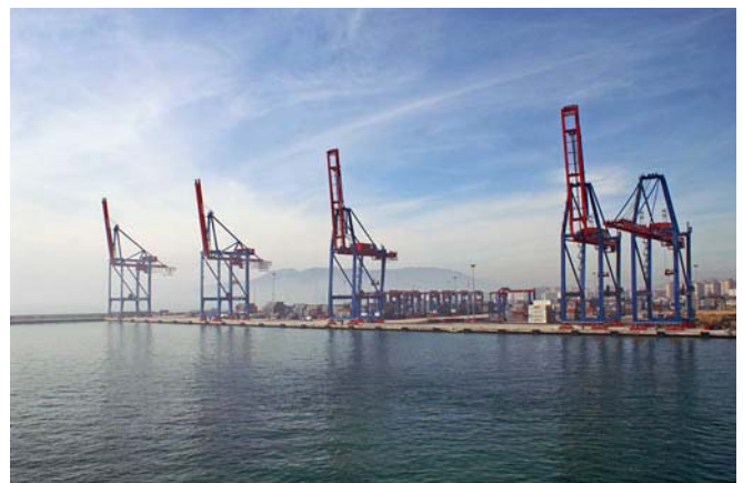
Wharf 9—Container Terminal
