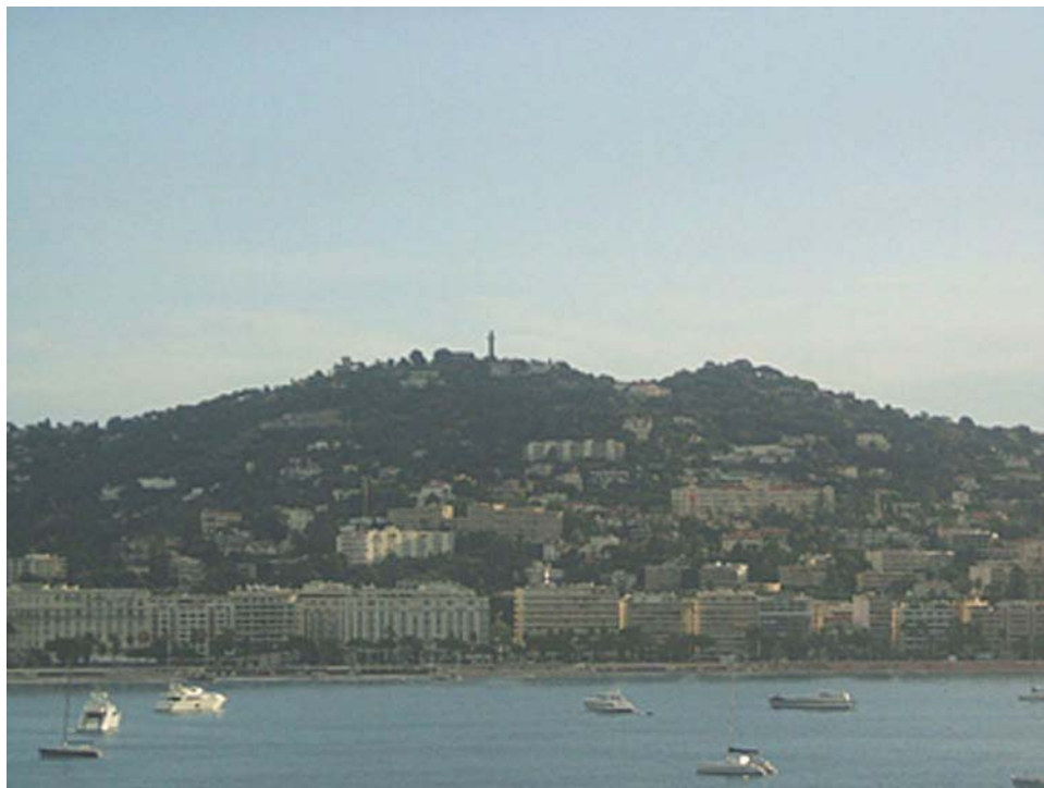
Cannes—Standpipe on Super-Cannes
