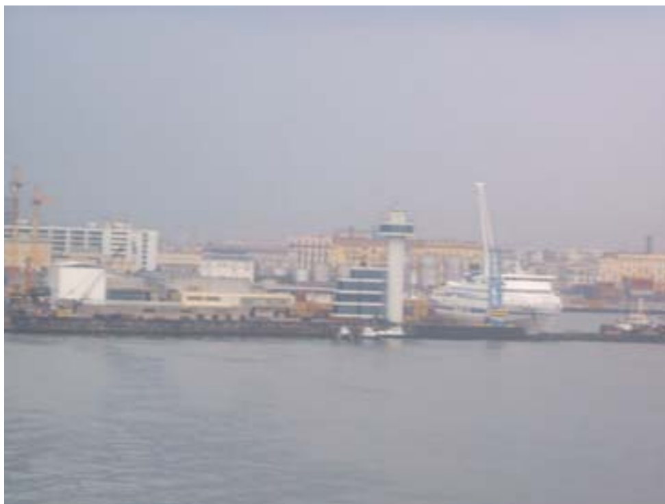
Napoli—Harbor Control Tower
