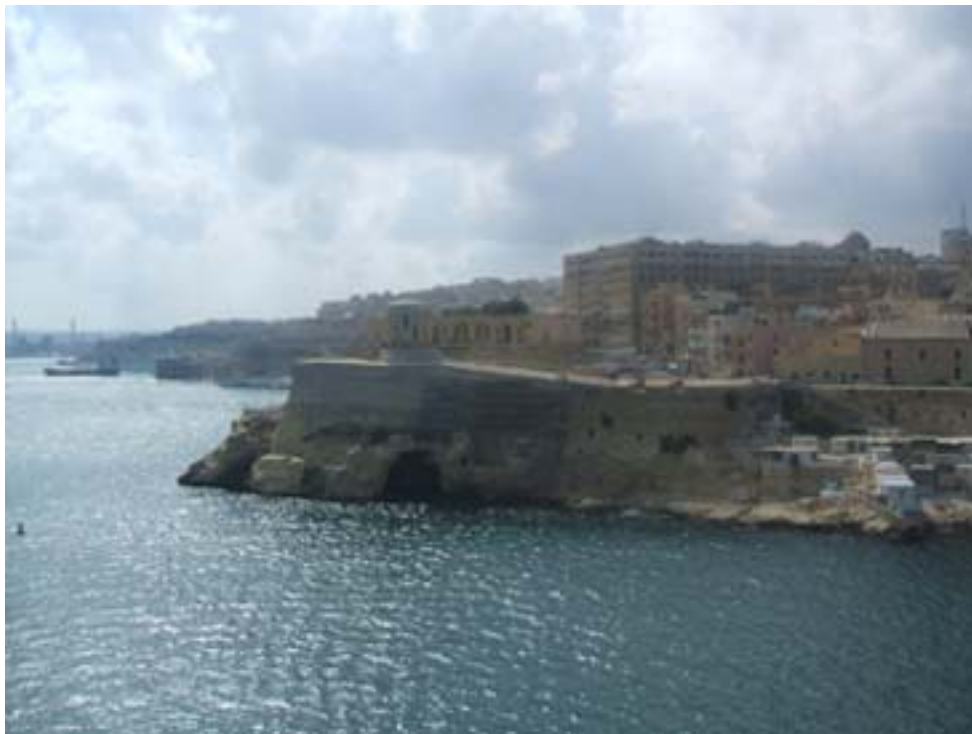
Valletta—Bell tower on Ponta ta L'Imgerbeb
