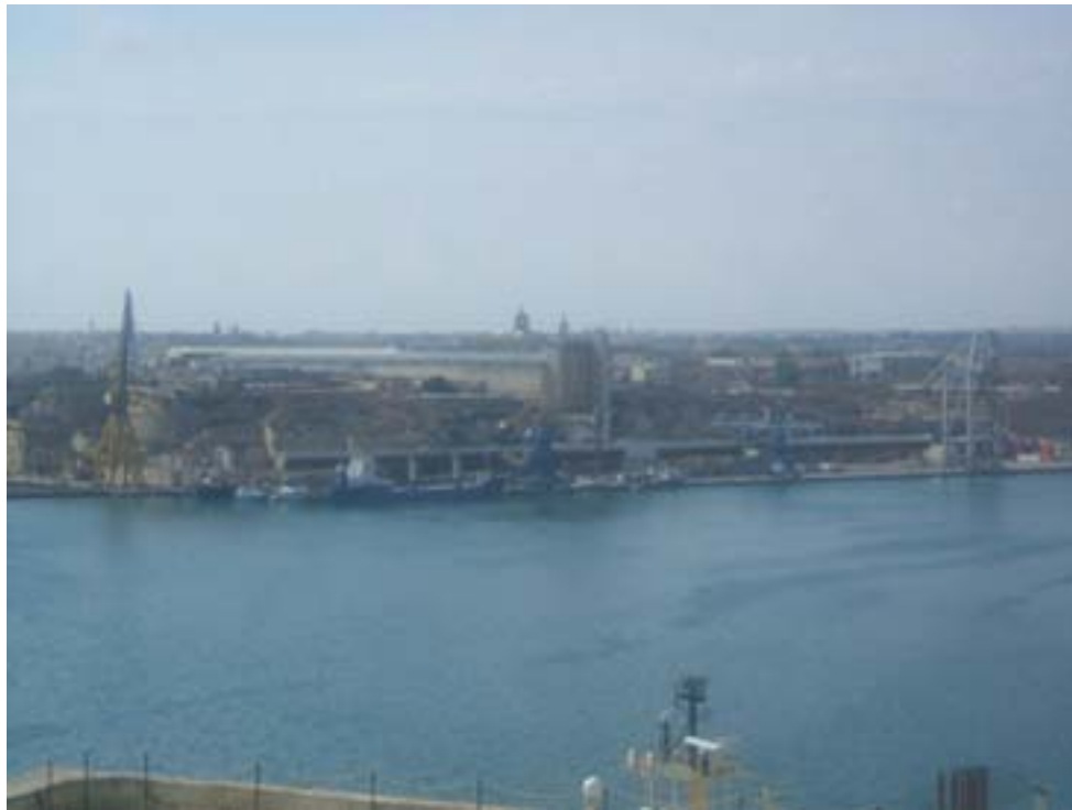
Valletta—Magazine Wharf (left) and Laboratory Wharf Container Terminal (right)
