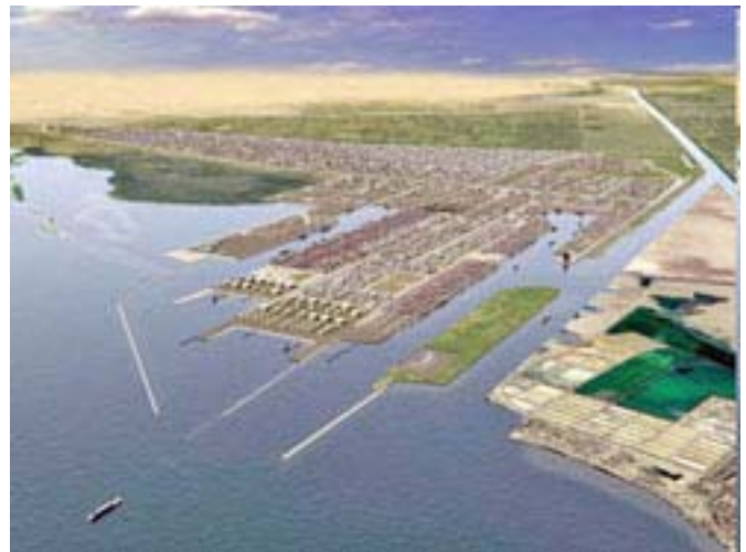
Port Sa'id (aerial view)
