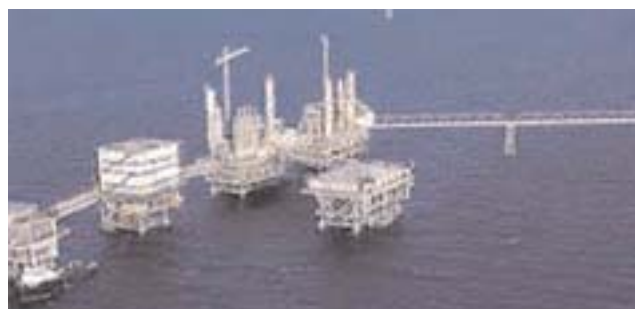
Production platform located in Ardjuna Oil Field
