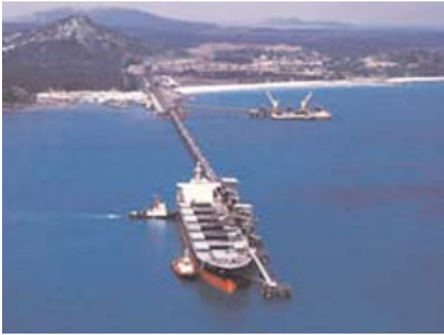
North Pulau Laut Coal Terminal
